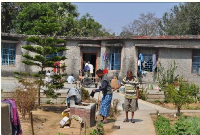
the new well
